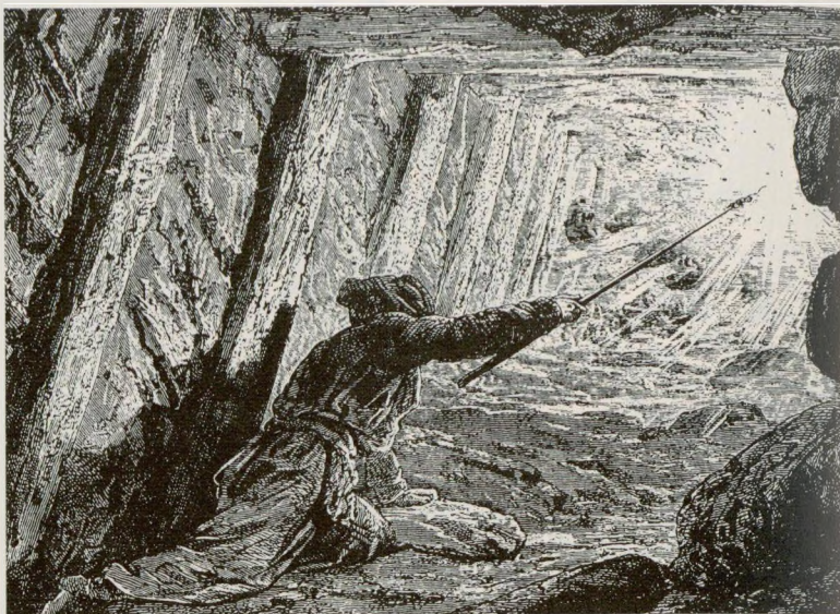
Fig. 3. Fireman igniting firedamp. (From Singer, C. J., Holmyard, E. J., Hall, A. R., and Williams, T. I.: A History of Technology . Oxford, The Clarendon Press, 1958, vol. 4, p. 92. By permission.)
