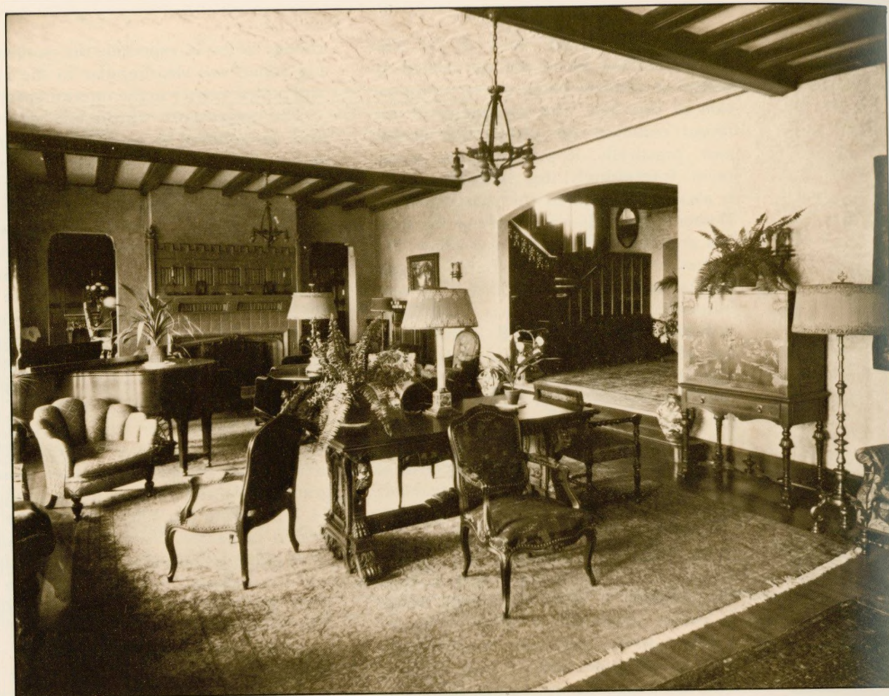
15. Living room, manor house. Photograph taken circa 1927.
