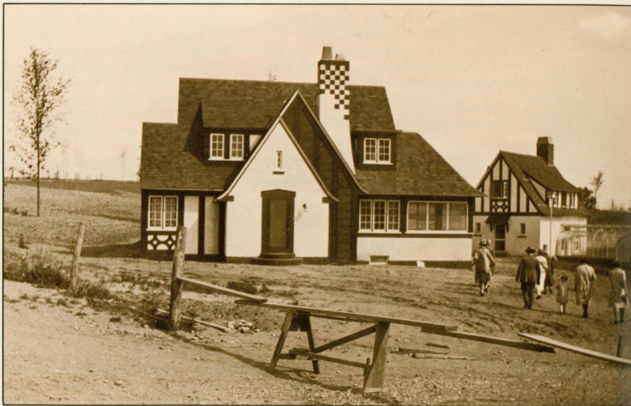
13. Caretaker's house during construction. Photograph taken 1926.
